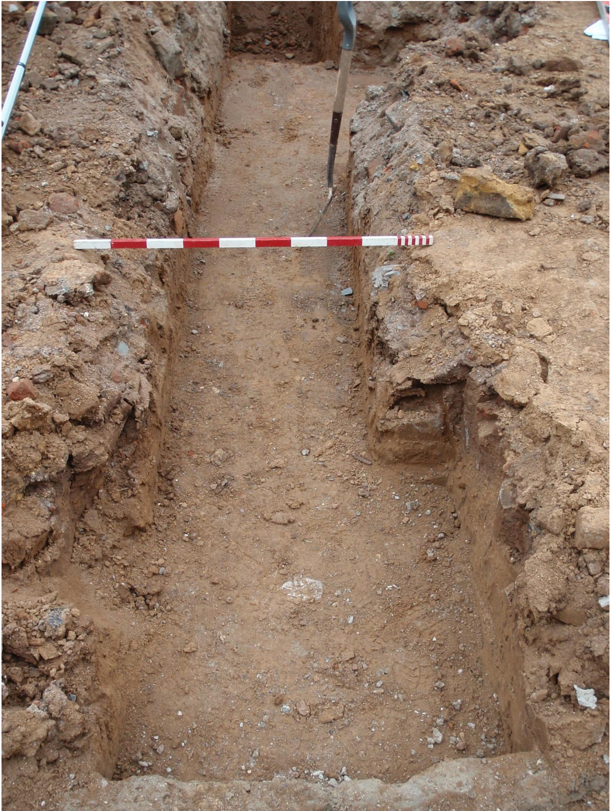
Plate 4. Foundation trenches facing north east
