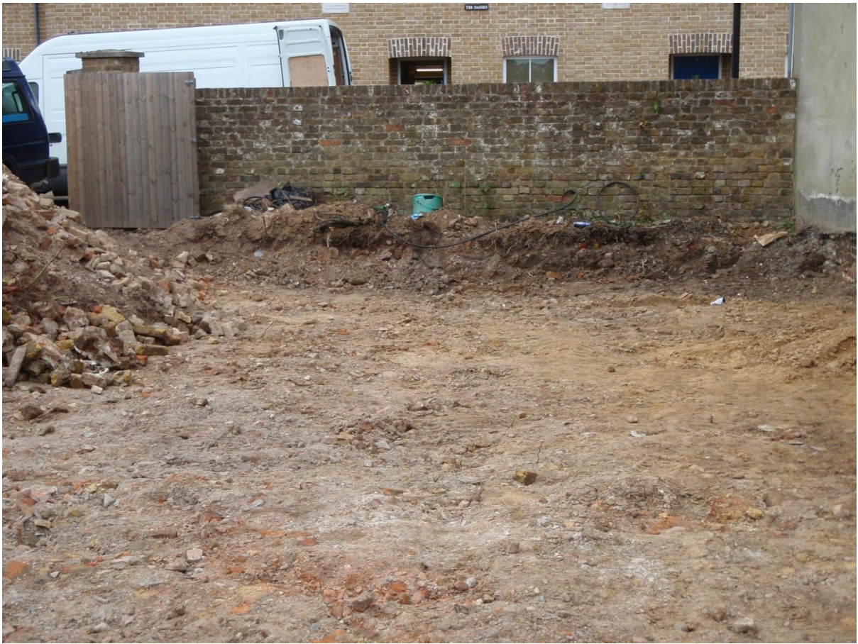
Plate 2. General view of site prior to ground works facing east
