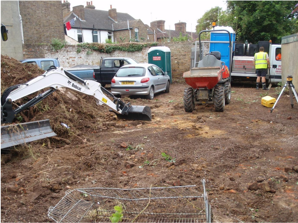
Plate 3. The site prior to ground works facing south west
